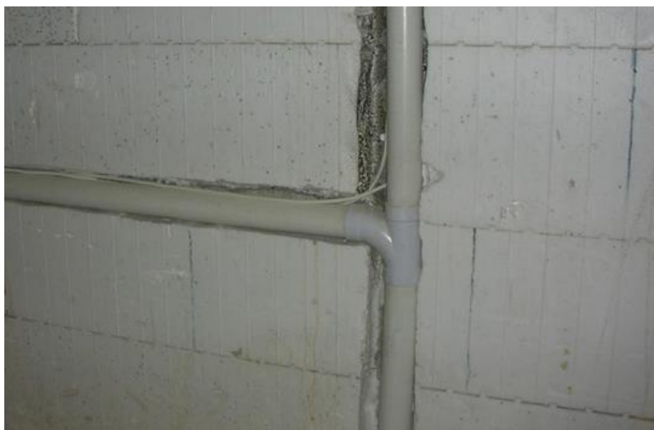
Recessed Pipe or Conduit (max 40mm)
