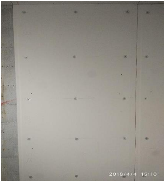
Wallboard with metal fixings 15/board
