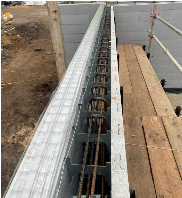
Reinforcement & Lintel Section
