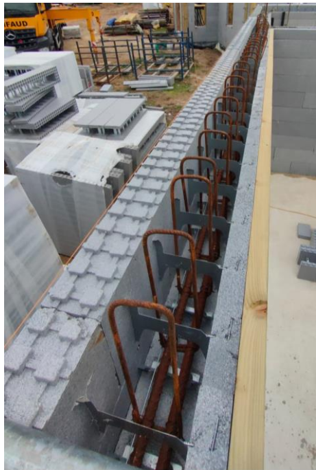
Reinforcement on Lintel Section
