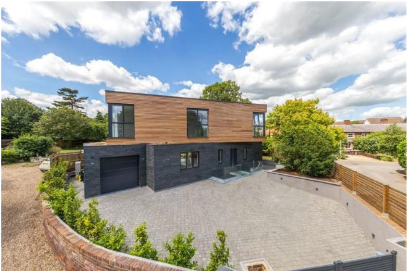
Timber Cladding with Stone Tiled walls
