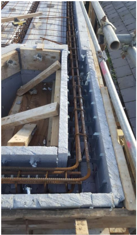
Reinforcement in Corner Section
