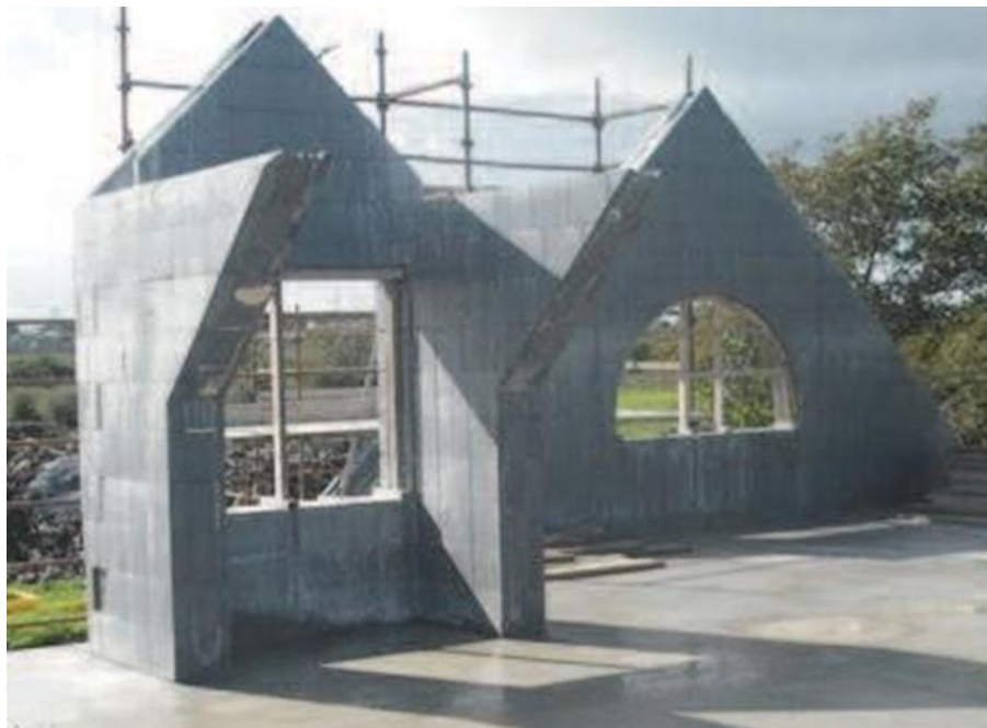
Dormer Window & Arched Window Photo
