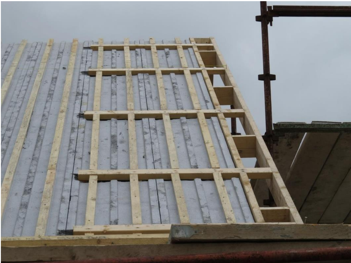
TR29a - Option A - Timber Ladder Gable End
