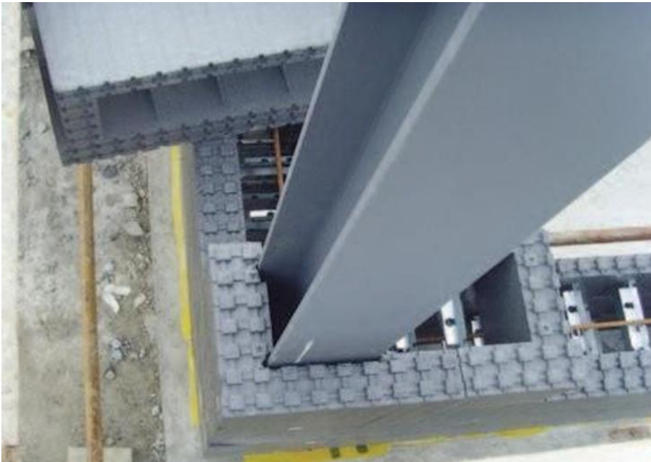
Wrapping a structural steel Photo
