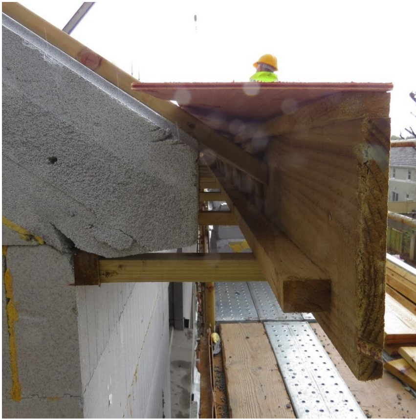
Facia & soffit Detail
