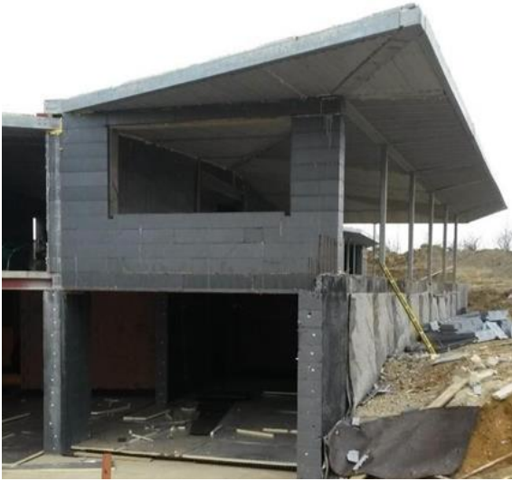
Multi Faceted roof with large overhangs
