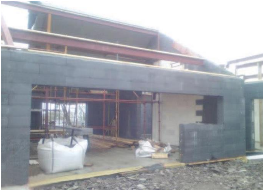
Long Span Window Photo
