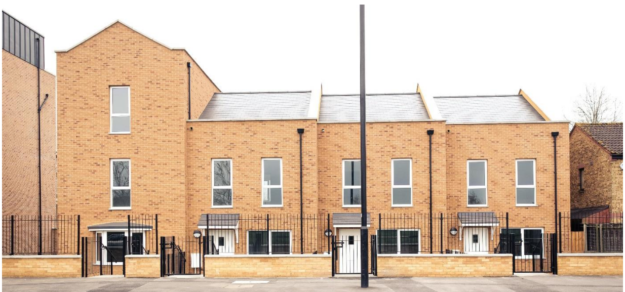
Brick Slip Finish to Apartment Block and Town Houses
