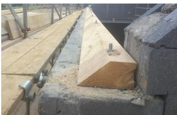
Installation/Fixing Chamfered Wall Plate
