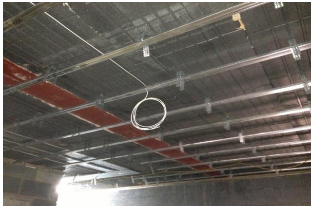
Suspended ceiling showing service void
