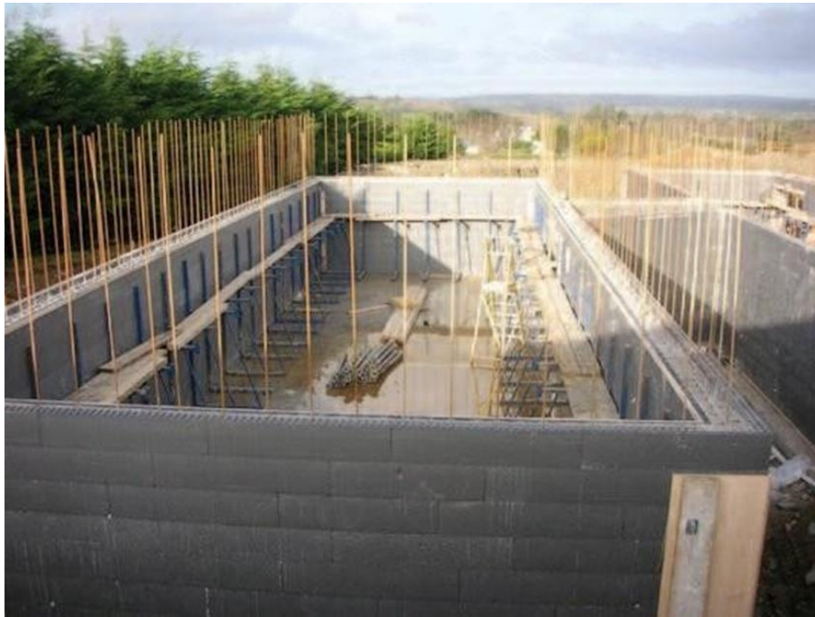
Standard basement construction
