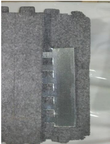
Fixing flange exposed through block
