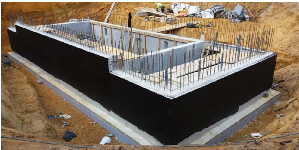
Lower basement showing initial tanking layer
