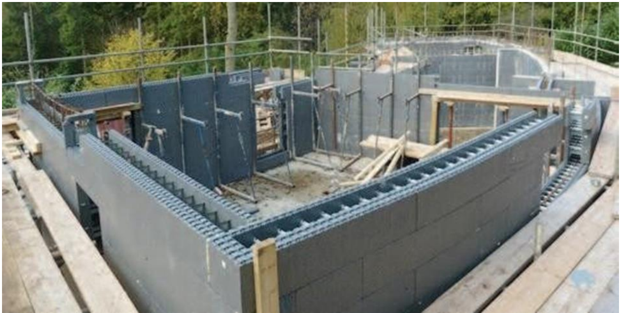
External Curved Wall Construction Photo
