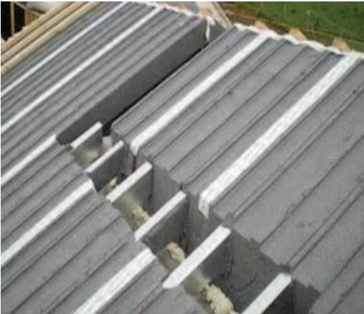
Void in Panels For Fire Batt infill
