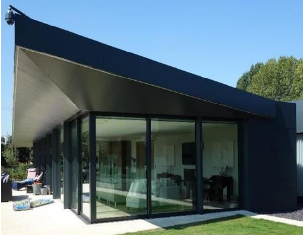
Multi Faceted roof with large overhangs
