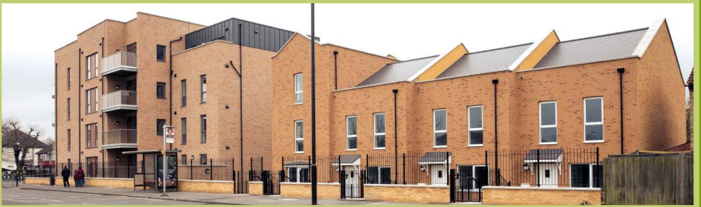
Terrace of 4 houses & 4 storey apartment block + basement
